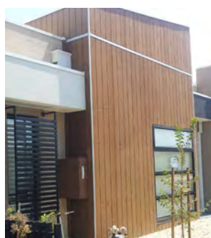
4 MONTHS: The board shows signs of lightening.
