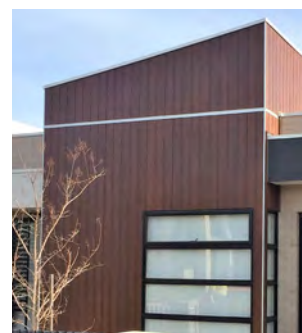
COMPLETE: After 3 coats the timber is restored and is now UV protected. Maintain the stain over time as per product directions.
