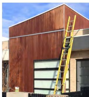
CLEANING: Wash the boards with a deck cleaner and a firm brush.
